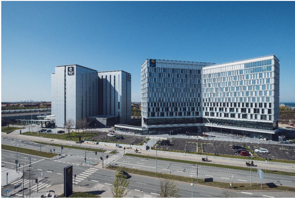
Clarion Hotel & Comfort Hotel next to each other at Copenhagen Airport
